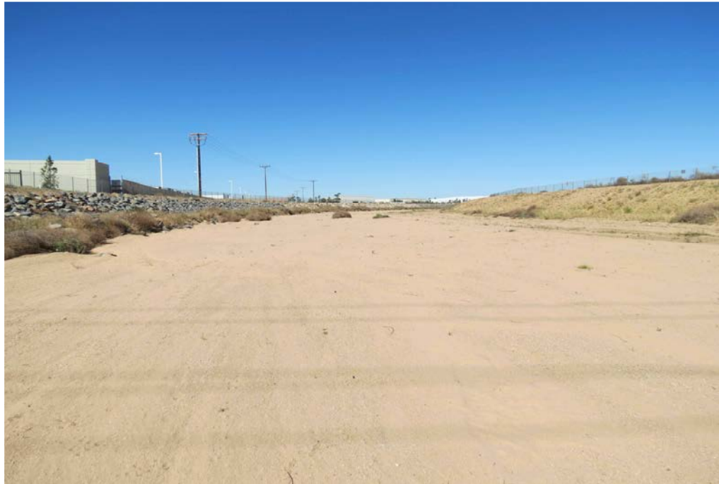
Photograph 2: Photograph depicting the Perris Valley Storm Drain.
