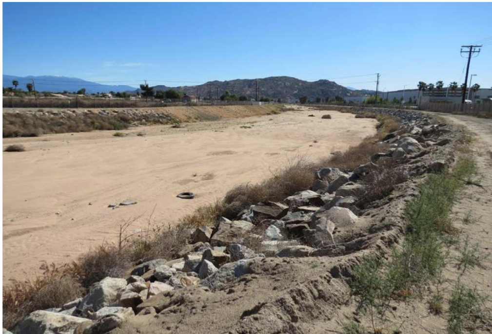
Photograph 1: Photograph depicting the Perris Valley Storm Drain.
